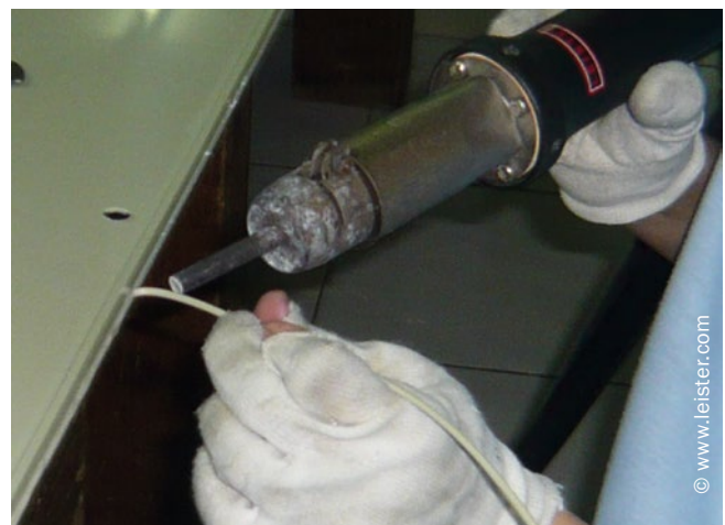
Figure 4: Hot-gas fan welding with circular welding rod
